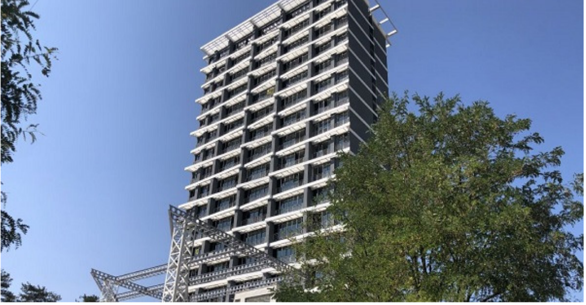
FINDIKKULE RESIDENCE Konuralp / Düzce (19 floors - 121 flats) Reference Yapı Fire Installation Projects and Contracting.
