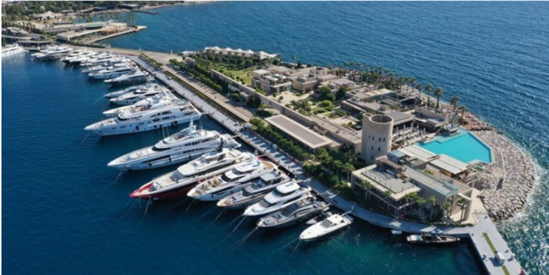
YALIKAVAK MARINA / BODRUM Fire installations and ventilation systems improvements commitment.
