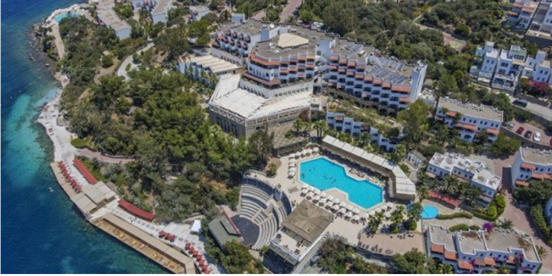
HILL SIDE HOTEL Gündoğan / Bodrum / MUĞLA Alarko Holding Infrastructure steel pipe (3.000 m.) manufacturing.
