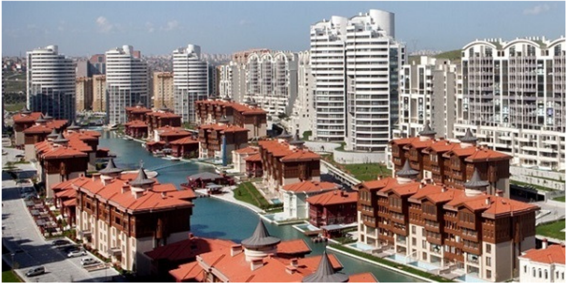
BOSPHORUS CITY Halkalı / İstanbul Sinpaş GYO Cihan Cons. Residence (3,000 flats) Mechanical Installation Site Supervisor.
