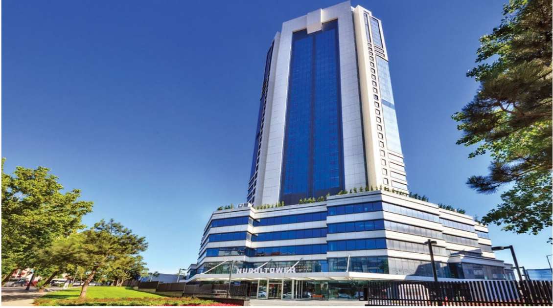
NUROL TOWER EOFİS FLOOR (150 offices) Şişli / İstanbul NUROL GYO Mechanical Installation Project and Contracting.
