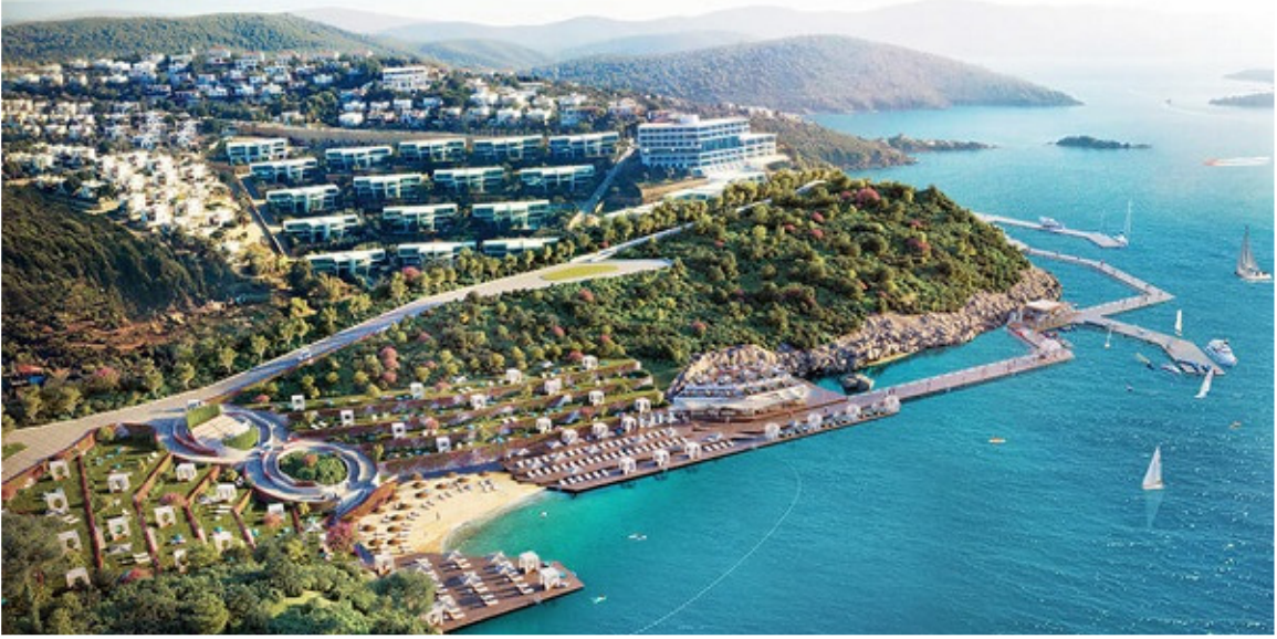
THE HOUSE RESIDENCE Bodrum / MUĞLA (194 villas) Helis Yapı Mechanical installations consultancy.
