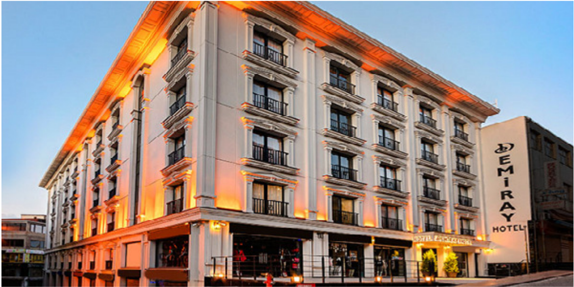
DEMİRAY (5*) HOTEL Sirkeci / Istanbul (120 rooms) Mechanical Installation project and contracting.
