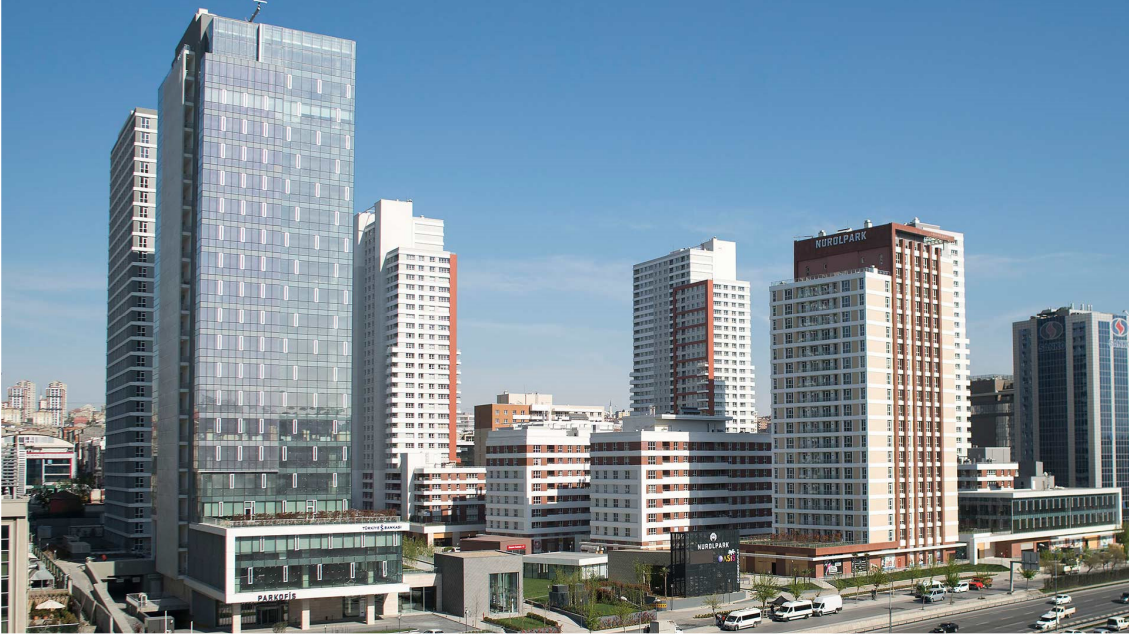
NUROL PARK EOFİS FLOOR (80 offices) Başakşehir / İstanbul Nurol GYO Mechanical Installation Project and Contracting.
