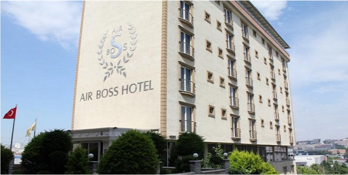
AIR BOSS HOTEL Basın Expres / İSTANBUL İzgün Turizm Additional floor mechanical installations project and contracting.
