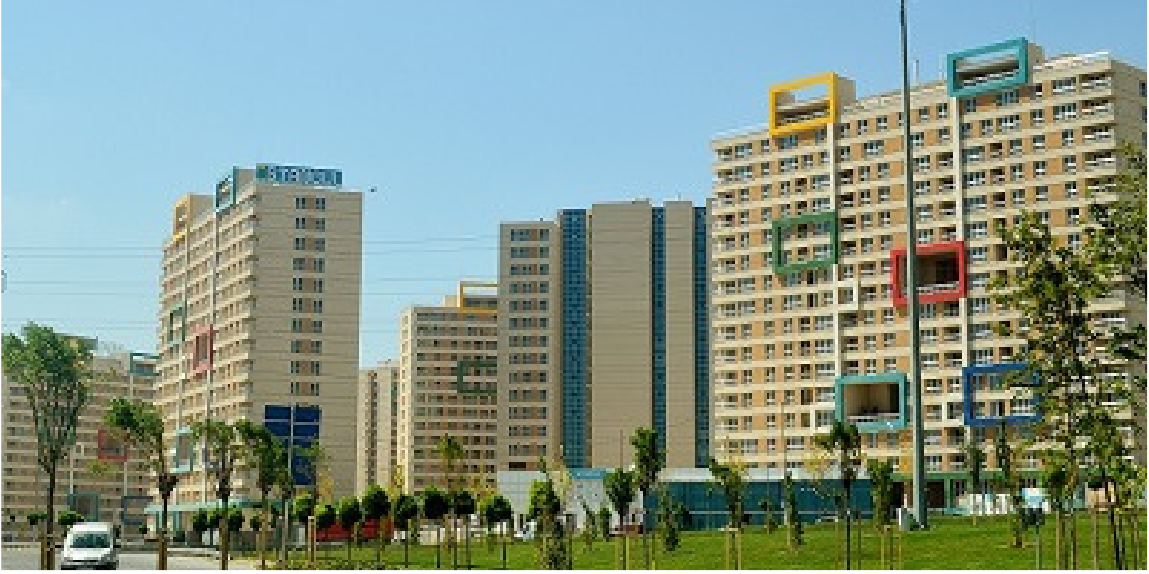
ONE ISTANBUL Emlak Konut Yeni Dođuř İnřaat Housing Social Facility (1.180 flats) Mechanical Installation Group Chief.
