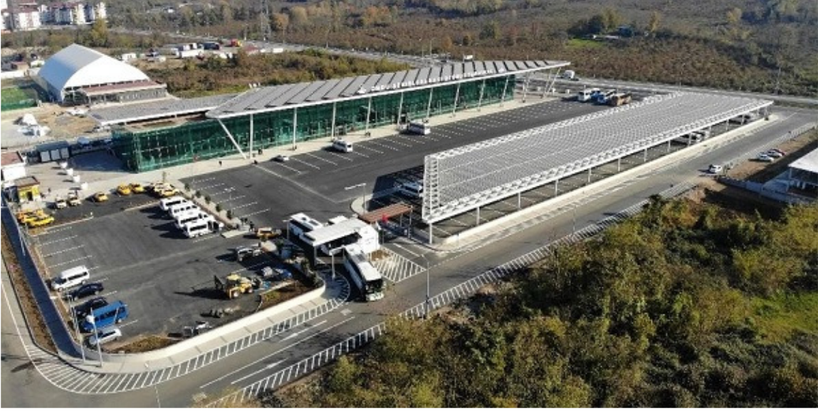
ORDU TERMINAL Merkez / Ordu OBB Gothic Architecture Terminal Building (4.000m 2 ) Heat Pump Mechanical Installation Projects.
