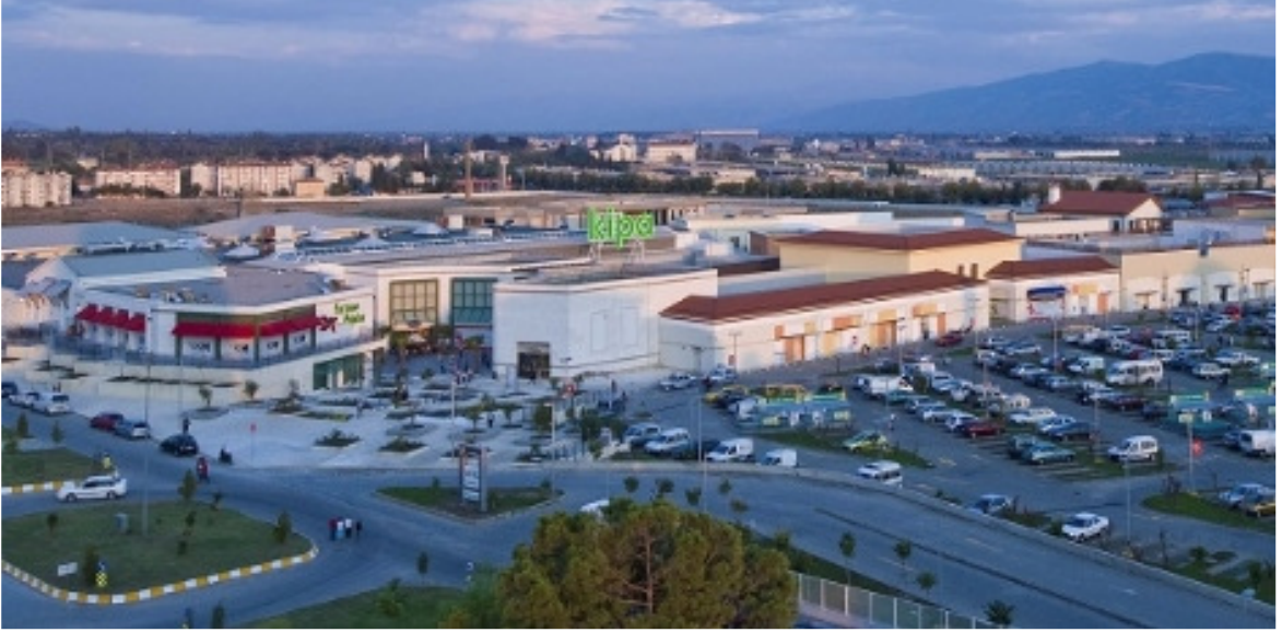
FORUM AYDIN Center / Aydın Multi Turk Mall – ERBA İnşaat AVM (80.000m 2 ) Mechanical Installation Control.
