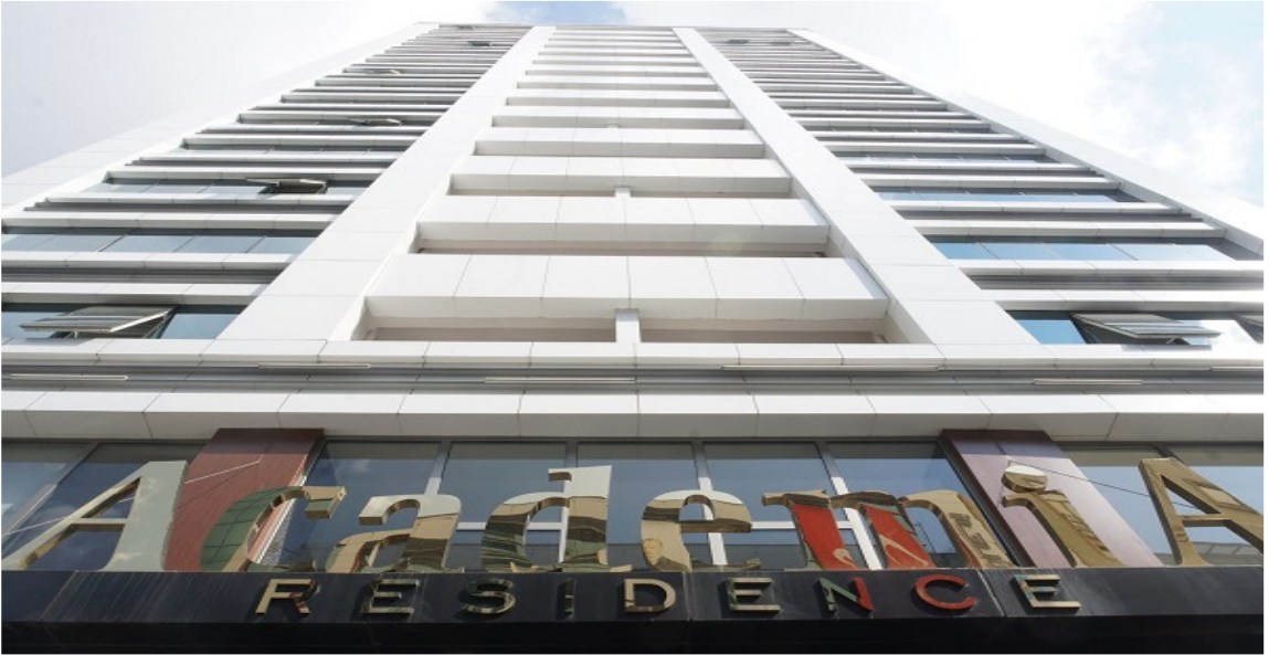
ACADEMIA RESIDENCE Kağıthane / Istanbul Petra Yapı Residence (18 floors – 108 flats) Mechanical Installation Control and Renovation.
